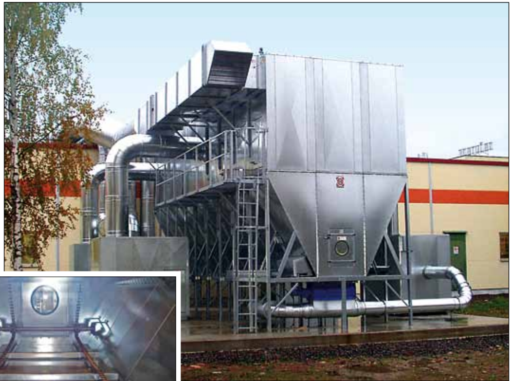
The photo to the left shows the inside of an Aagaard chain filter hopper.
