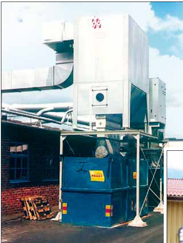
Aagaard rotary valve filters on standard Aagaard container stands.
