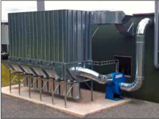
Aagaard bag-emptying filter with hopper-mounted explosion relief doors (ATEX approved) and steel bins at Swedish kitchen manufacturer – air volume 45,000 m 3 /h.
