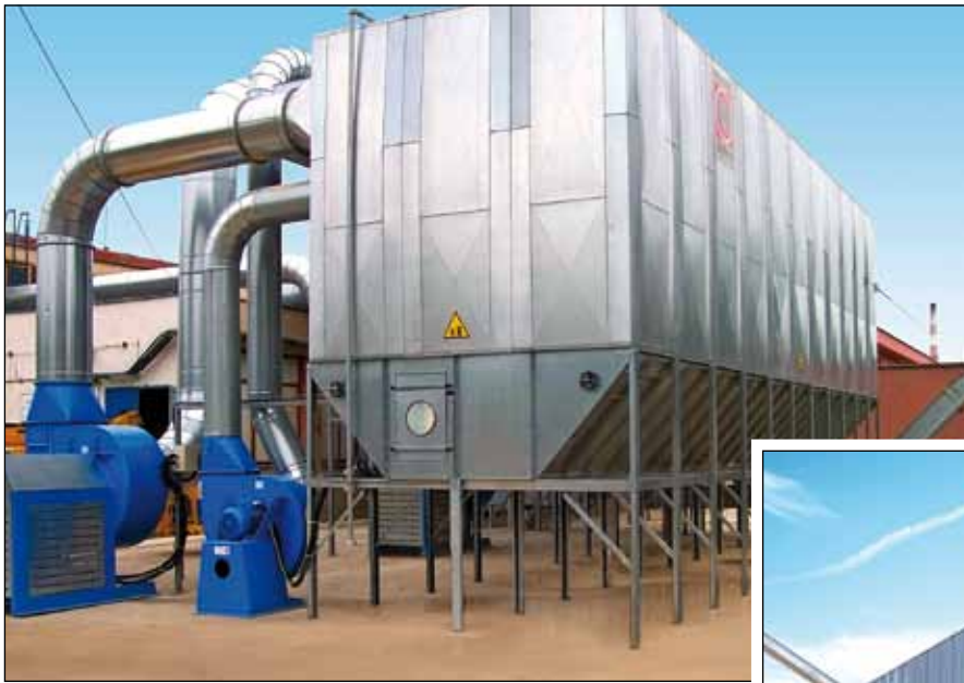
Aagaard chain filters at a furniture factory in Klaipeda, Lithuania and Swedwood's laminated wood factory in Tikhvin, Russia respectively.
