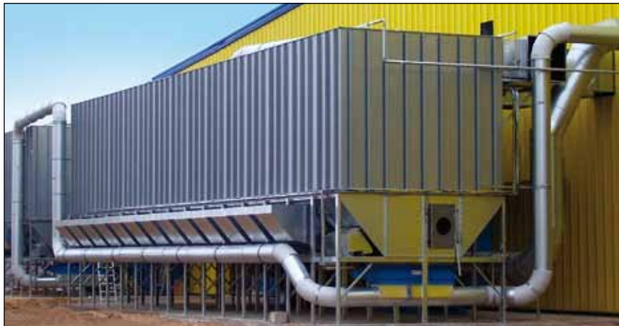
Aagaard chain filter with hopper-mounted explosion relief doors at a factory in Belarus – air volume 250,000 m 3 /h.
