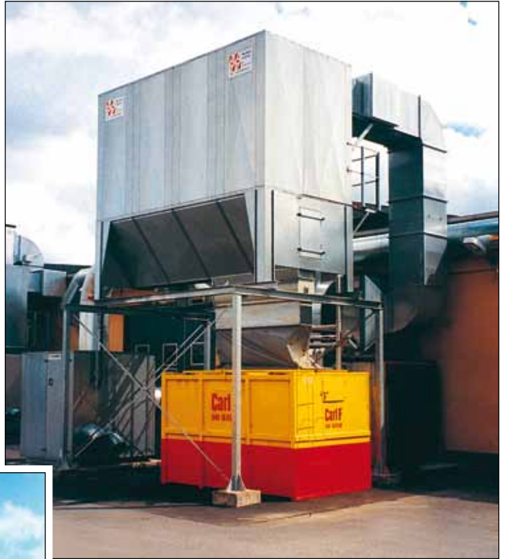
Aagaard rotary valve filters on standard Aagaard container stands.
