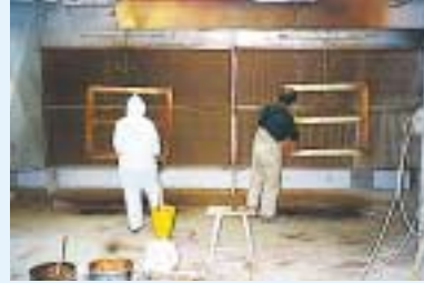
Spray painting of windows/doors.
